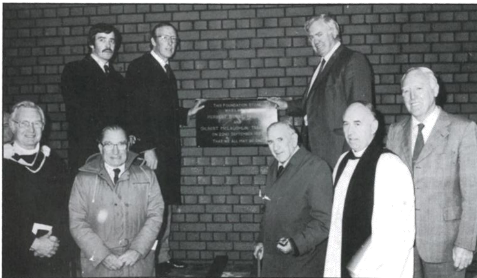
New Beginnings: Laying of foundation stone - Y.M.C.A. New Building Drumahoe 22nd September 1984
